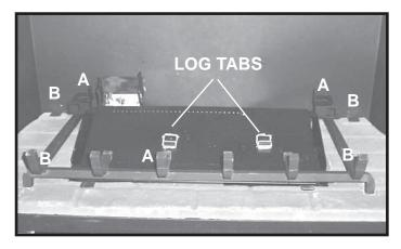
**STEP 1:** Remove metal grate supports (A) and refractory tabs (B) by using a back and forth motion until the tabs break free. Metal tabs and supports are needed for shipping only. After removing the tabs and supports, the grate should fully rest on the base refractory.
